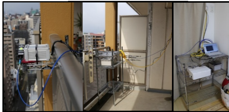
Fig. 4 Photographs of the compact MAX-DOAS instrument installed at Yakuin, Fukuoka.
